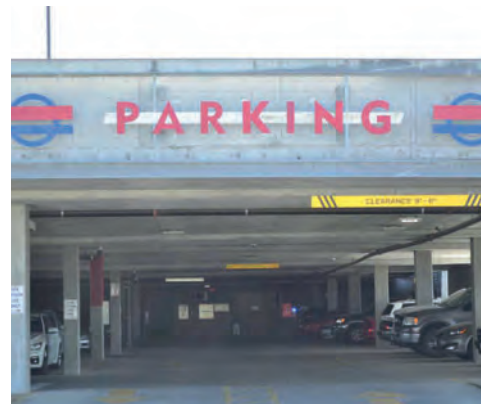
Type 12 Parking Structure Identification (Wall Mounted)
