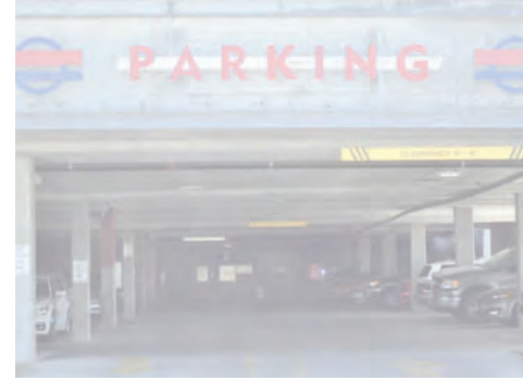
Type 12 Parking Structure Identification (Wall Mounted)
